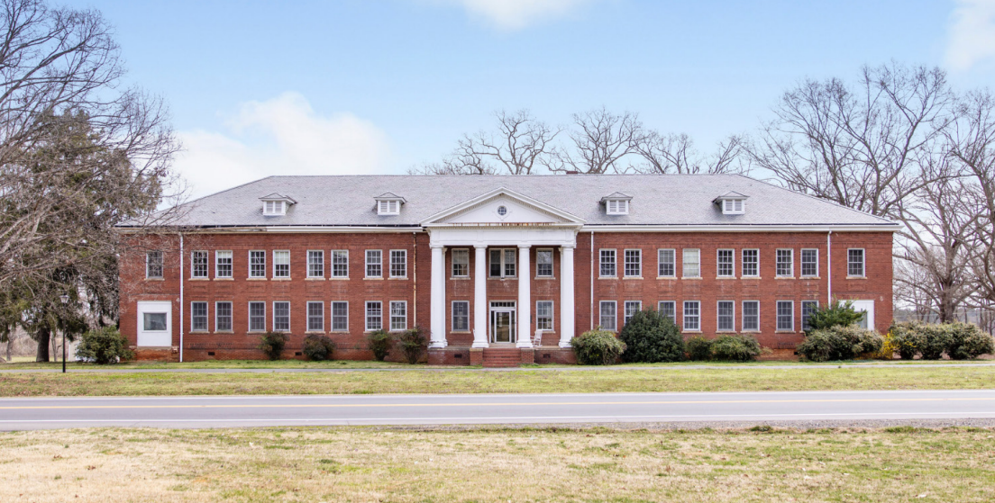
The site of the future Troutman Life Center
